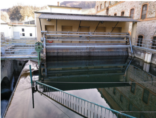
Current photograph of the small dam at Pioppe di Salvaro.
